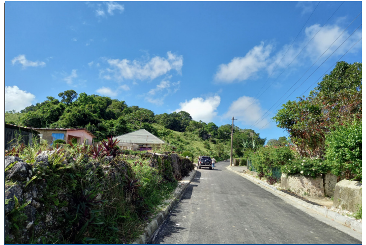
Epworth Main Road, after rehabilitation.
