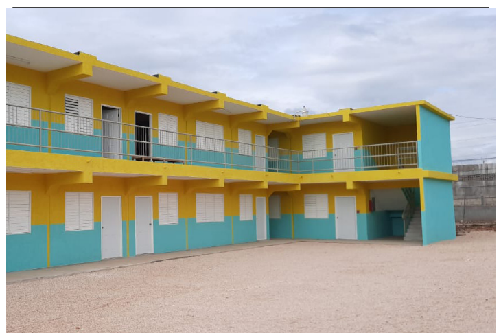
Marlie Mount Primary newly constructed 10-classroom block with an 8-seater sanitation block.
