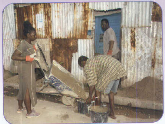
Construction activities underway
