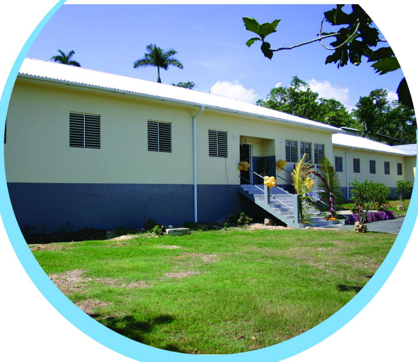
Homestead Place of Safety after rehabilitation.
