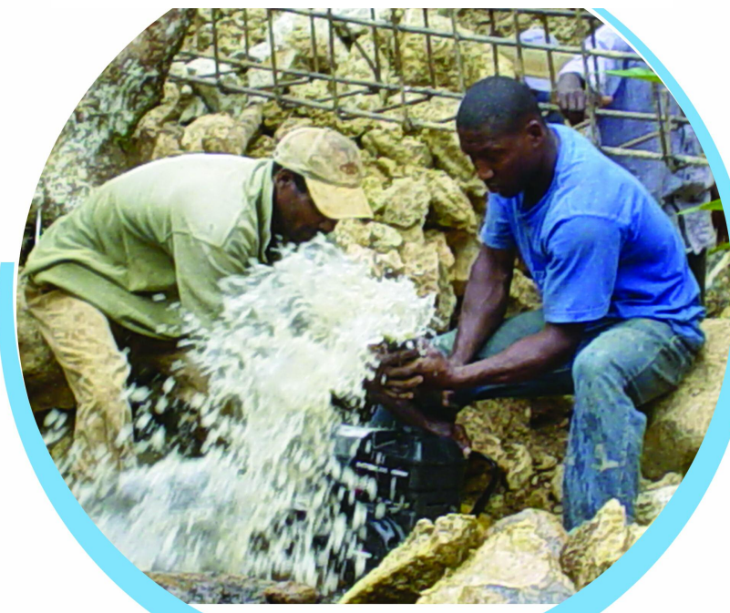
Workers at Pedro River draining the catchment area to cast the dam wall
