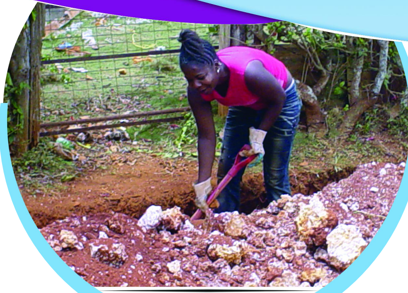
Community labourer working on the Rowlandsfield Water Supply project
