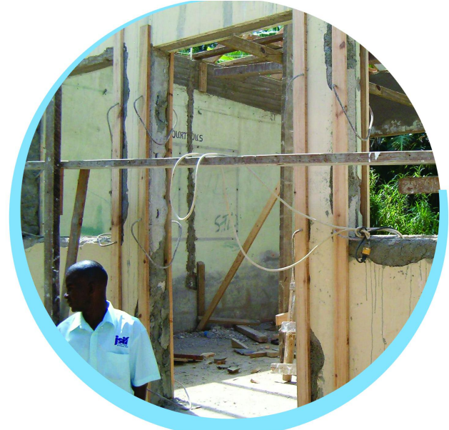
Work in progress at Homestead Place of safety.
