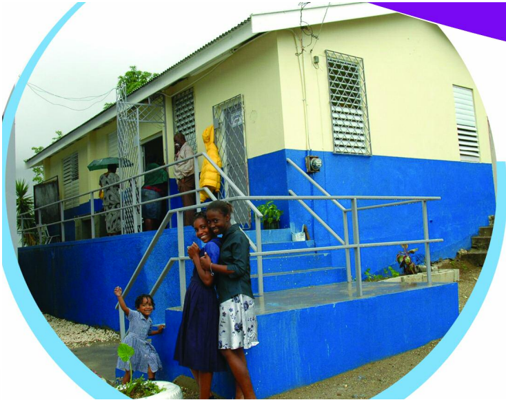
Beneficiaries of the Craighton All Age School in front of the newly finished building.
