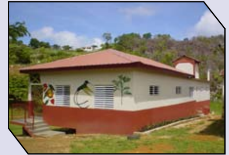
The newly construction Medina Basic School in Manchester
