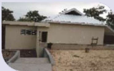
The newly constructed Arcadia Basic School nears completion
