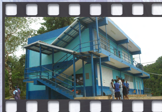
The finished classroom block at the Rock Hall All Age School
