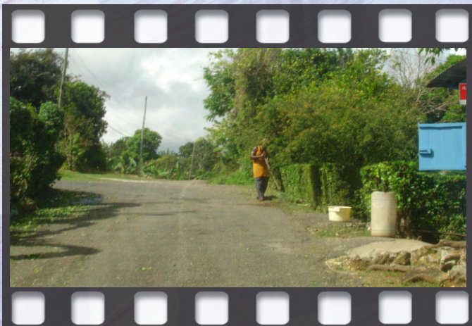
Maintenance Activities on the Grande Hill to Packi River Road
