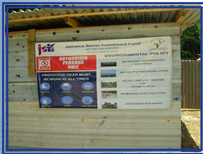
An environmental and safety sign mounted at a project site
