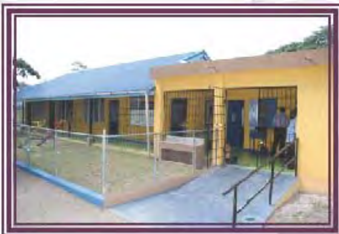
Construction and equipping of the Islington Early Childhood Institution in St. Mary was completed at a cost of $39.431 million. The school was built to the standards of the Early Childhood Commission's new approved basic school model and boasts computer systems, interactive white boards, projectors and pin boards, among other features.
