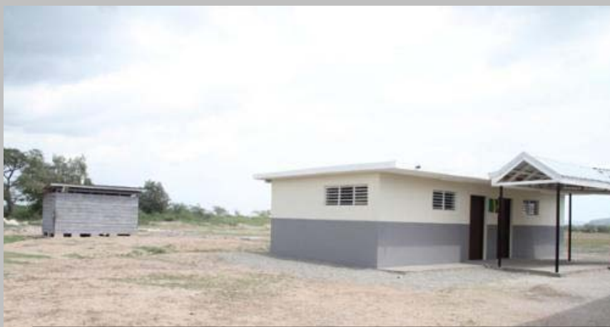
The sanitation block at Milk River Primary School in Clarendon stands in contrast to the old facilities in the rear. The Petro Caribe Development Fund (PDF) Schools Sanitation Project implemented by the Jamaica Social Investment Fund enabled the replacement of pit toilets in 26 schools which was funded to the tune of JMD$177.5 million.
