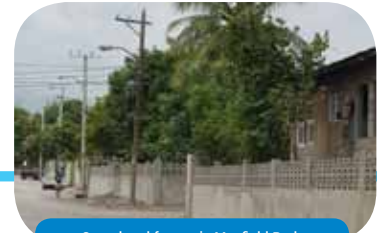
Completed fences in Maxfield Park
