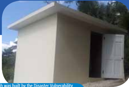
Seismic station at Mount Edgecomb in Westmoreland, which was built by the Disaster Vulnerability Reduction Project (DVRP), to house machinery which will monitor earthquake activity. This forms part of the net-work of monitoring stations which is being established across Jamaica
